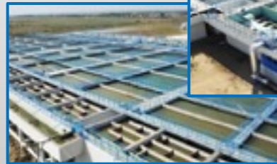
Flocculators & Sedimentation tank
