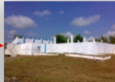
Clear water tank
