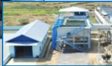
Low Lift Pump Station & Water tower
