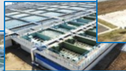
Rapid sand filter
