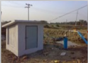
Pump House & Tube well
